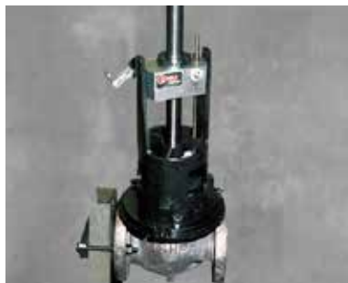
VM8000 Globe and Control Valve Repair
